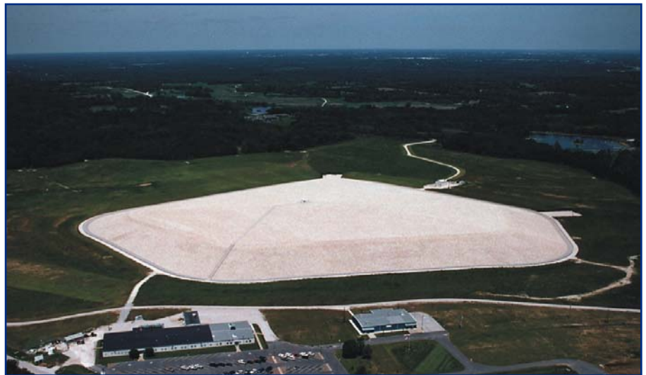
Weldon Spring Disposal Cell – September 2002
